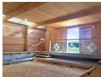
Tile protection shelter, Cleeve Abbey
