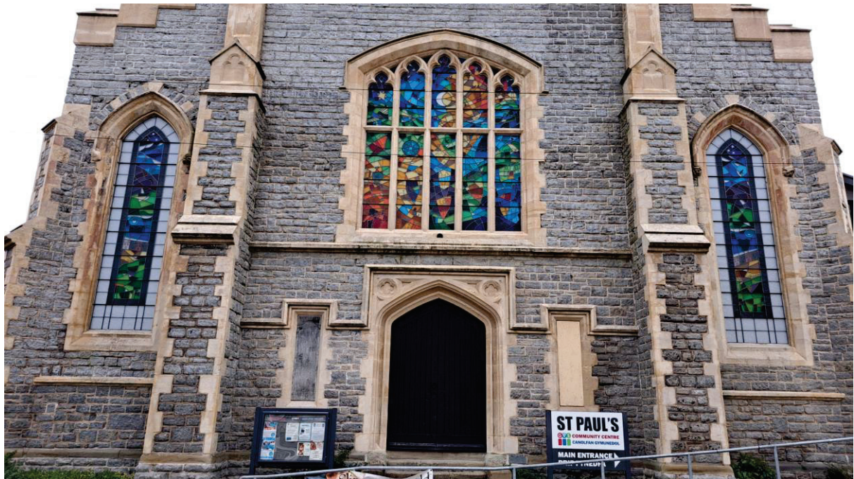
Completed main central window and side windows
