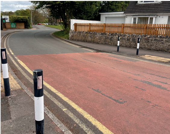
Poor pedestrian access along The Broad Shoard
